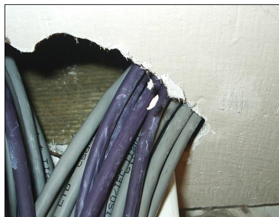
Asbestos insulation board (AIB)
