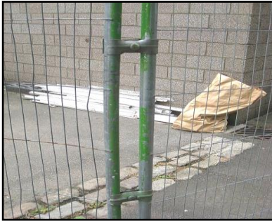
✓ Panels double clipped together
