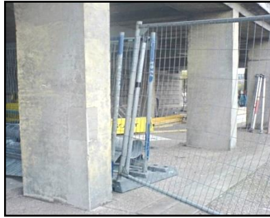
✗ Panels not double clipped to each other
