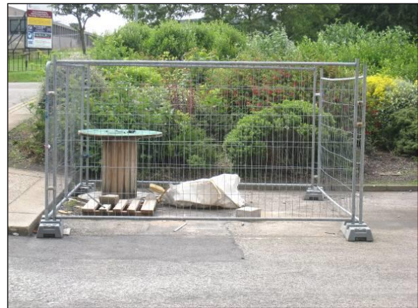
✓ Heras fencing put up around materials outside main site compound
