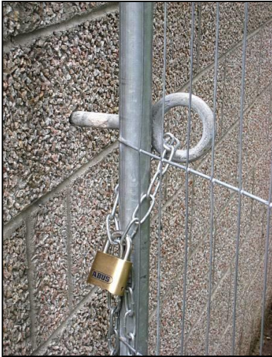
✓ Eyebolt, chain and padlock (best method)
