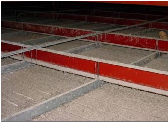
Sprayed asbestos
