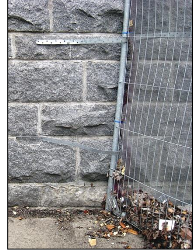
✓ Fencing straps screwed to wall
