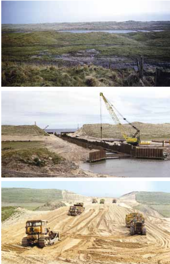
Figure 5.12 Pipeline laying at St Fergus Gas Terminal (Ritchie, 1997)
