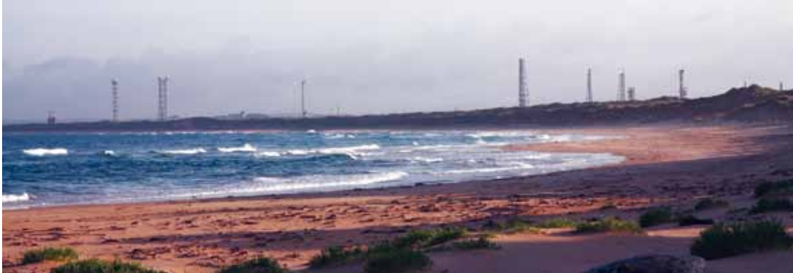
Figure 1.3 St Fergus Gas Terminal with its rural, coastal setting (Hay, I. 2007)
