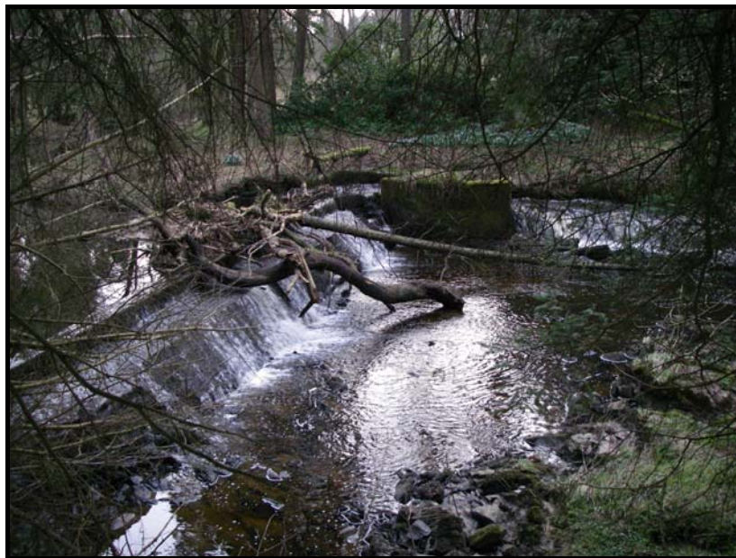
Plate XIX: Derelict weir on the Linhouse Water (upstream of a significant natural barrier)
