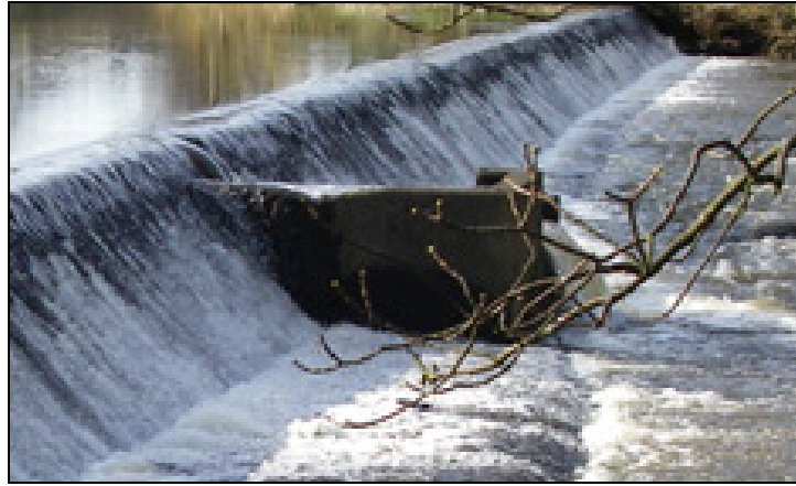
Plate V: Box-type fish pass at Mid Calder Weir (Plate III enlarged)
