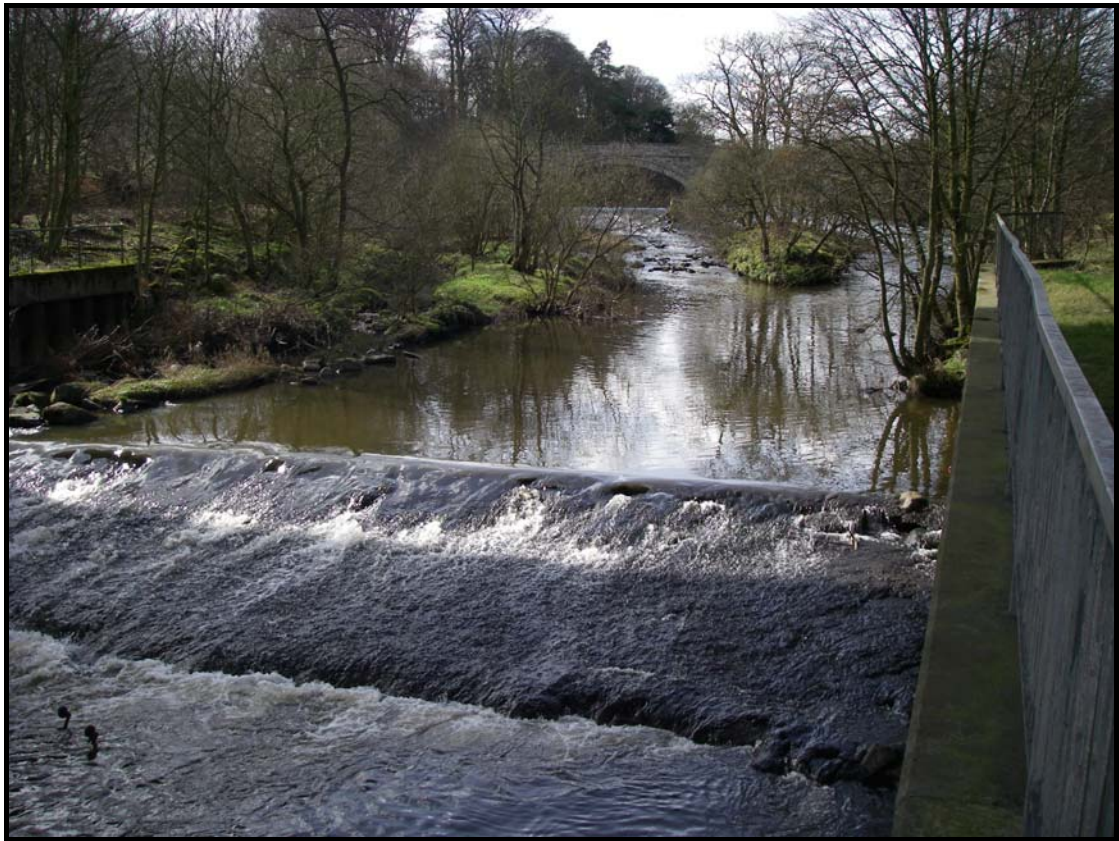
Plate XIII: Weir below Almond Valley Bridge
