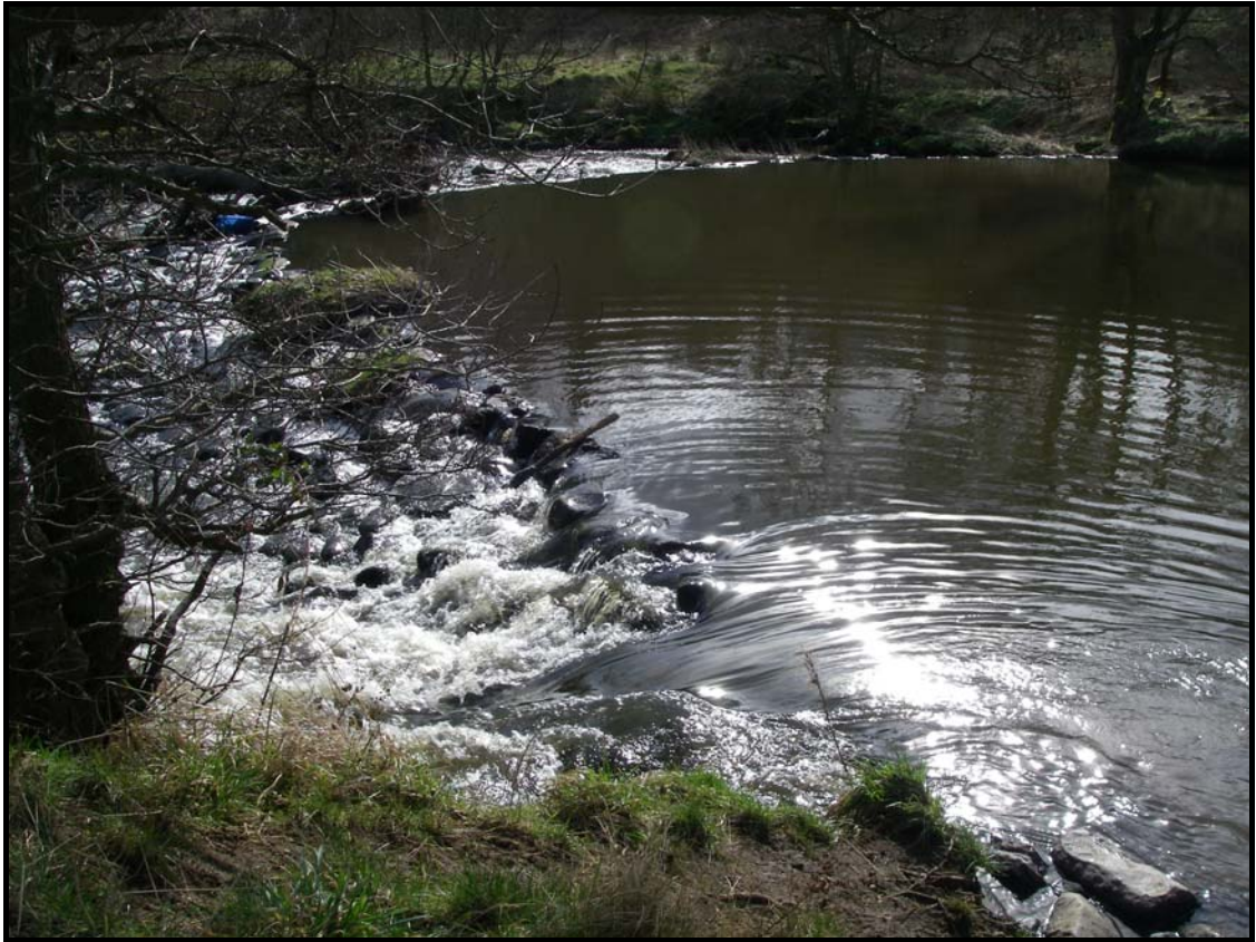
Plate XII: Curved, cobble weir also near the Rugby Club
