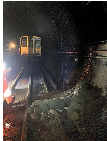
Augers within a tube railway tunnel after penetration, London, 2013. Source: RAIB, 2014.
