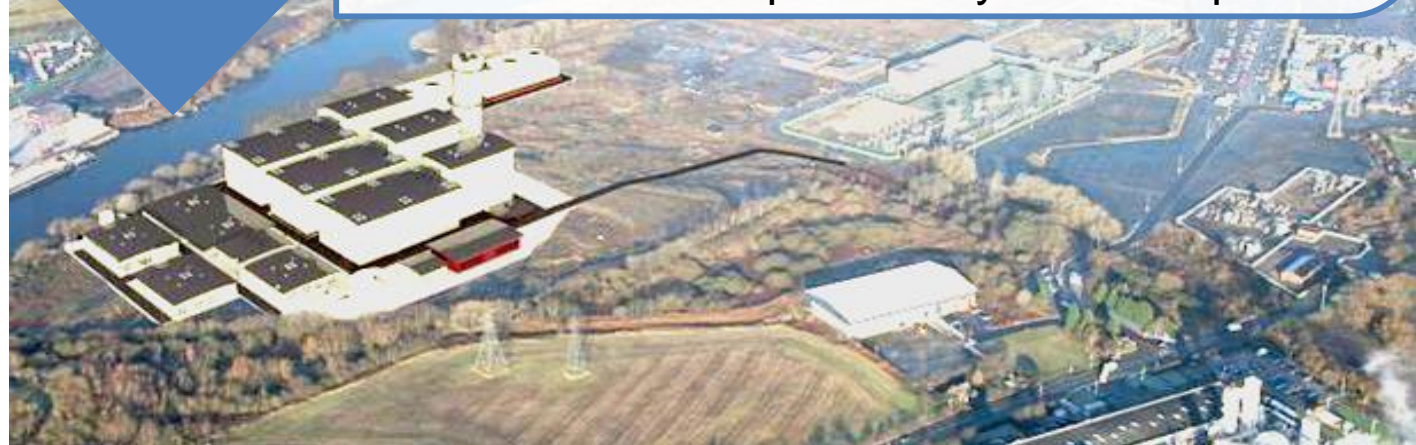
Trafford Power, the one & only new build CCGT Plant in the UK.
