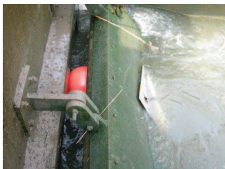
View from downstream (pet door is open)
